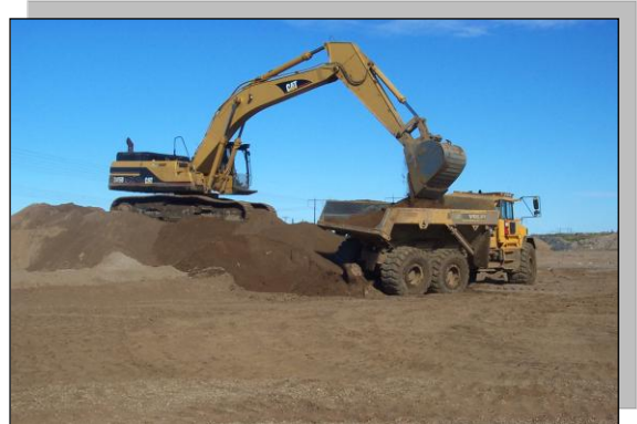
Poplar Creek Clean-Up & Stockpile of pit-run for processing
