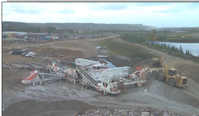
Suncor - Engineered Backfill
